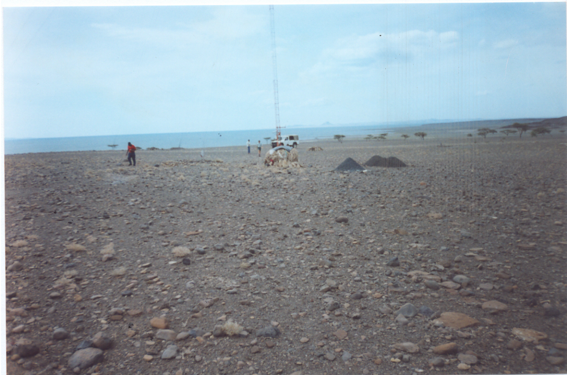
Plate 6: Lake Turkana Windpower mast at Loyangalani.
