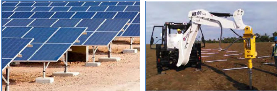
Figure 3-26 PV Module Foundation Establishment
