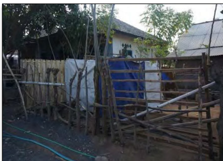
Figure 5-12 Water Hose for Water Connection from PDAM
