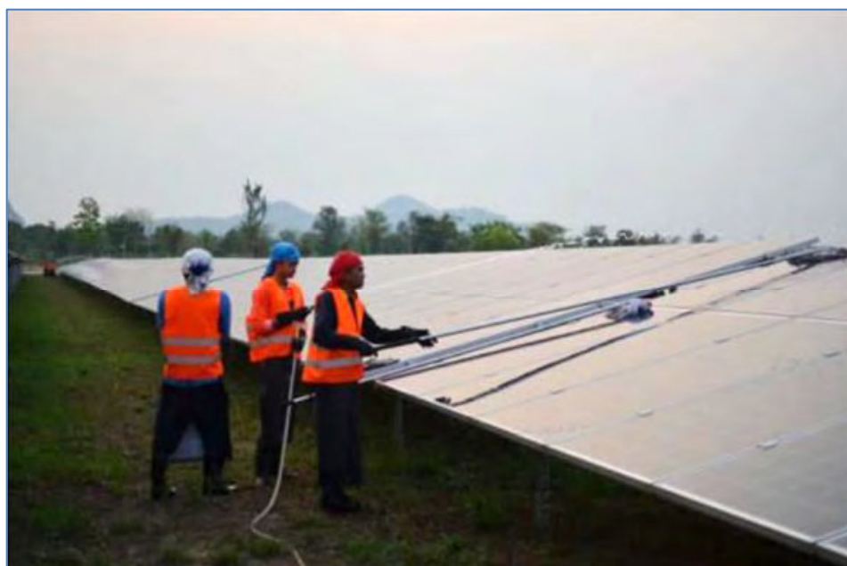
Figure 3-32 PV Module Washing
