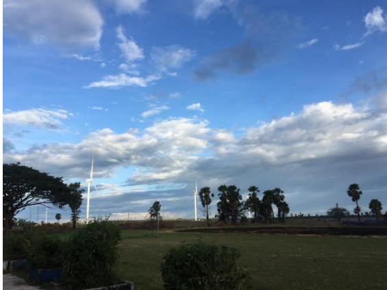
Photo 1. View of wind turbine generators from neighboring school
