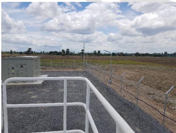
Photo 5. Wind turbines are fenced with locked entry
