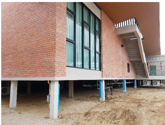
Photo 3. Back view of the main control building
