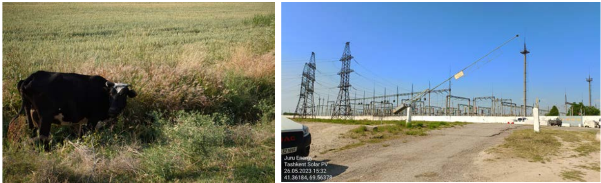
Figure 2-4 Pasture field within the BESS site (left) and the existing sub-station south-west of the area (right)
