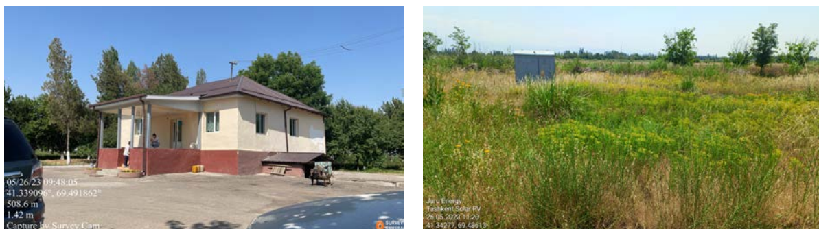
Figure 2-2 Uzsvtaminot administrative offices (left) and pump station (right) within the PV plant site
