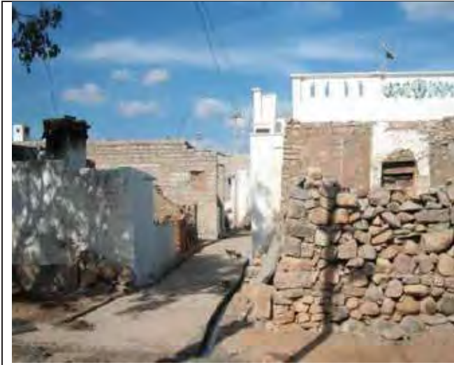
Picture of Open Drainage System in the Village of the study Area
