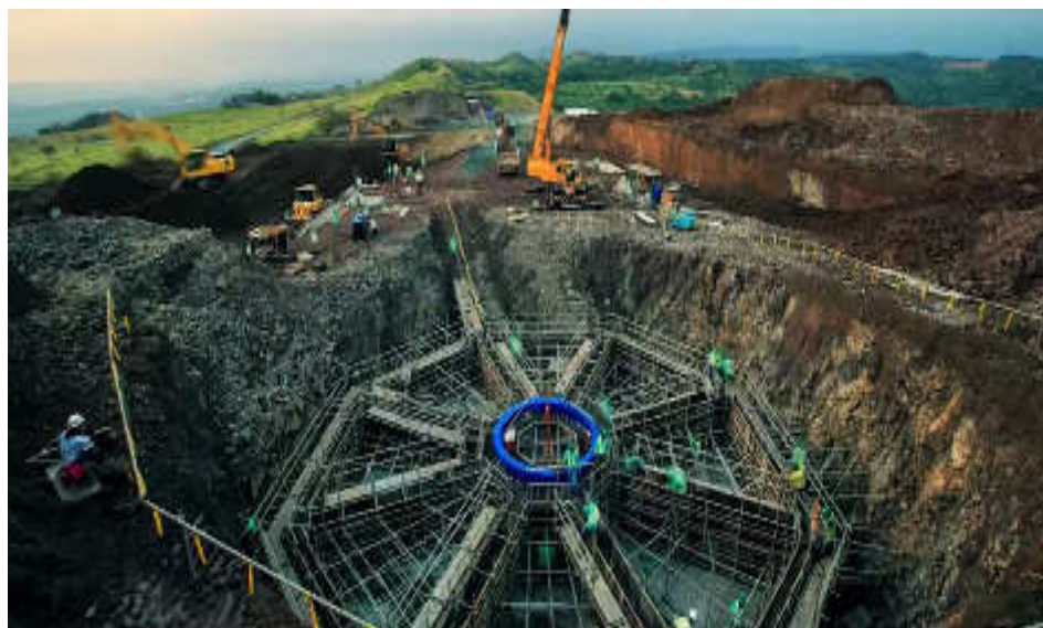
Figure 4-4 Example of WTG foundation type
