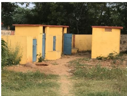
Separate toilet arrangements at Upper Primary School, Thumu Kunta
