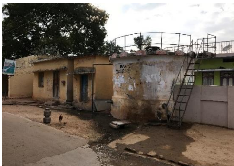
Above ground tank at Thumu Kunta village
