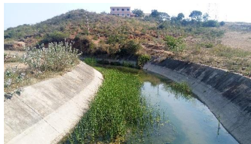
Irrigation Canal East of the Reservoir
