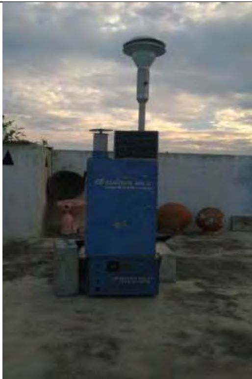
Joharapuram Air Quality Monitoring
