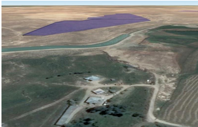
Figure 3: View of Omicron Erciş and Omicron Engil 208 Solar Power Plants from the nearest houses in the south-west
