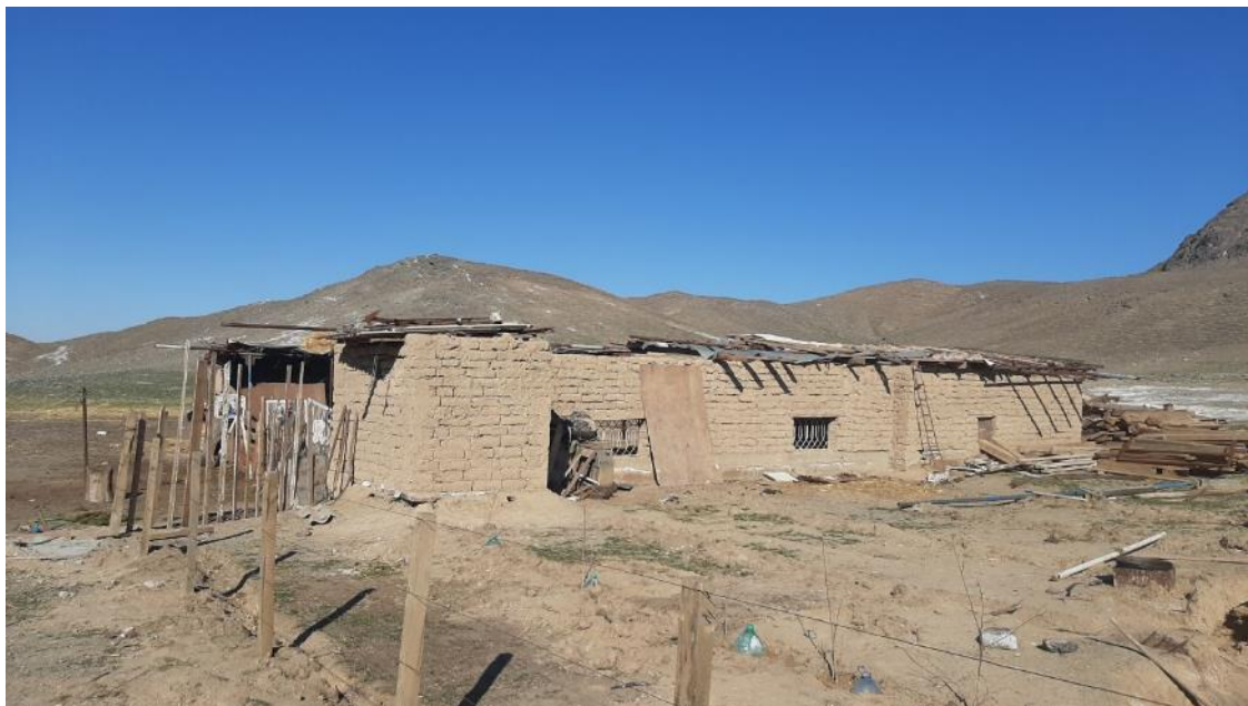
Figure 2-5: Herder Shelter within the Project Area
