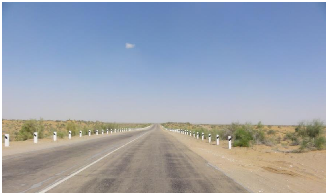
Figure 8-1: Road Condition A739 North of Zarafshan 116
