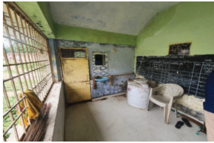
Toilet facility in PHC of Jakhan village
