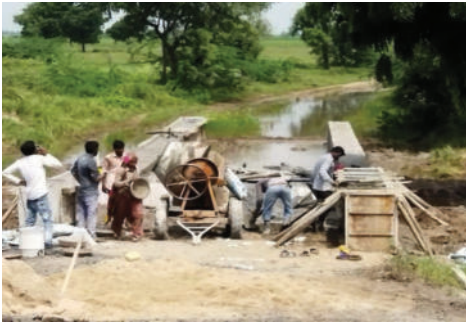
Approach road towards project site
