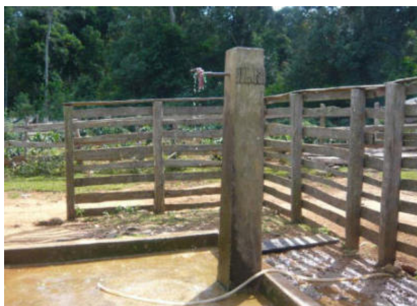
Gravity-fed water system in Prao Village
