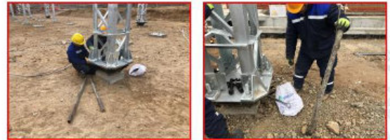
Torque wrench is using to tighten bolts around Switch portal frame
