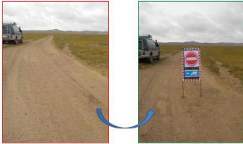
Installed Road Sign for Safe Driving
