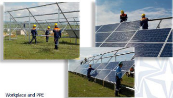
Workplace and PPE
