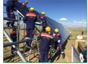
Workplace and PPE
