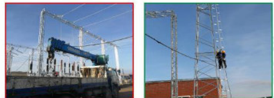
Crane boom is having danger to touch this 380V power cable ( Electrical risk hazard )
