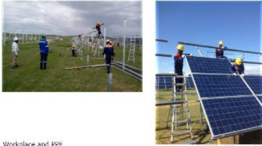
Workplace and PPE
