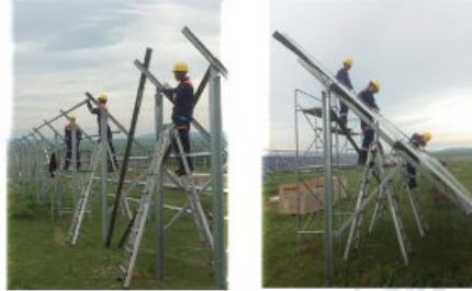
Workplace and PPE
