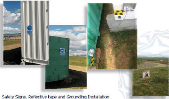
Safety Signs, Reflective tape and Grounding Installation
