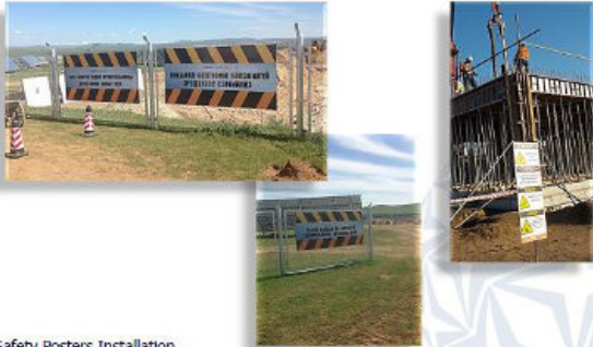
Safety Posters Installation
