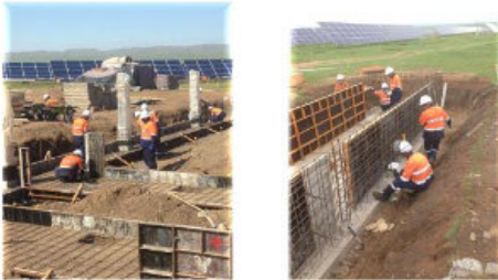
Workplace and PPE
