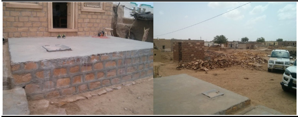
Figure 6.28 Water Tanks in Households
