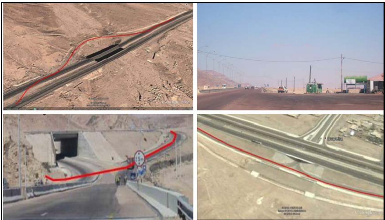
Figure 64: Bridges that will be Bypassed and the Bypass route and Other Obstacles in Place (utility lines)
