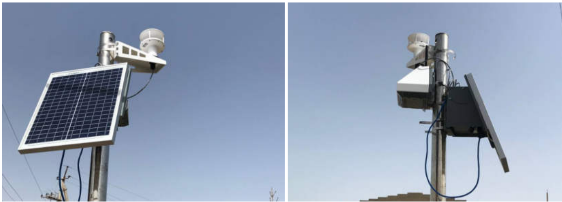
Figure 10: Air monitoring system at NA 1
