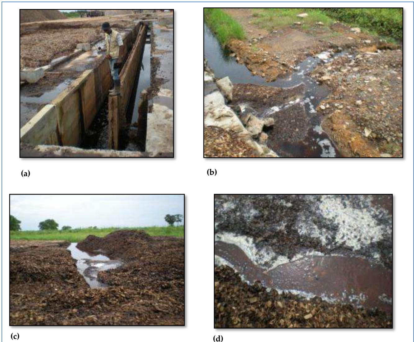
Figure 5-2: (a-d) storm water from piles of wood chips discharging into a nearby creek at the port of Buchanan
