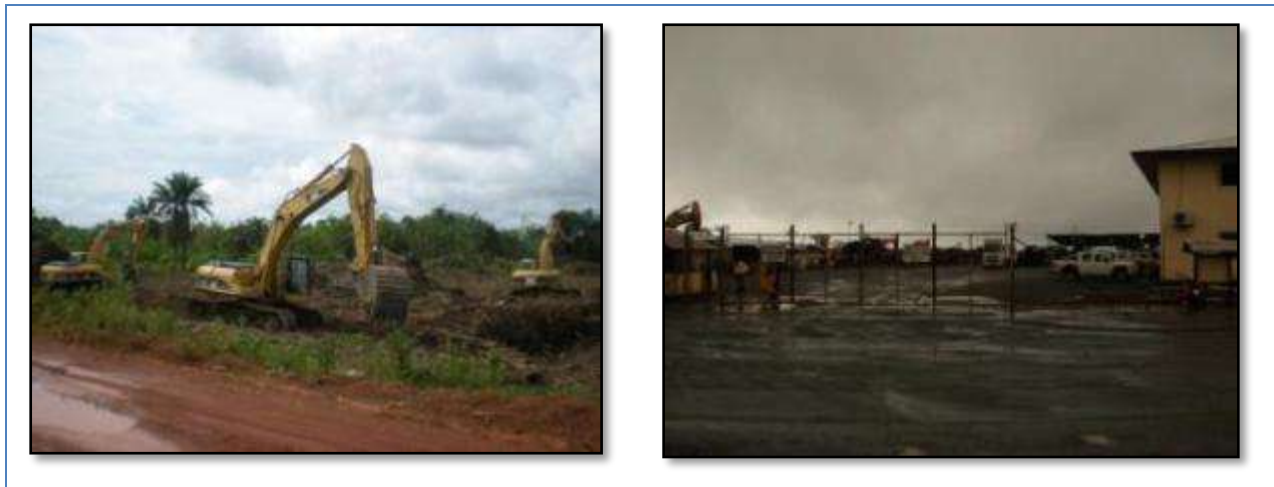
Figure 5-6: External view overlooking the project sites.
