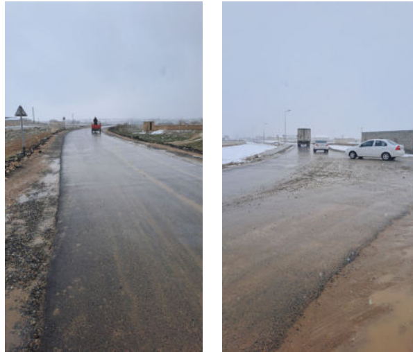
Figure 13-7 Municipal road nearby the 400 MW PV power plant and pooling station sites
