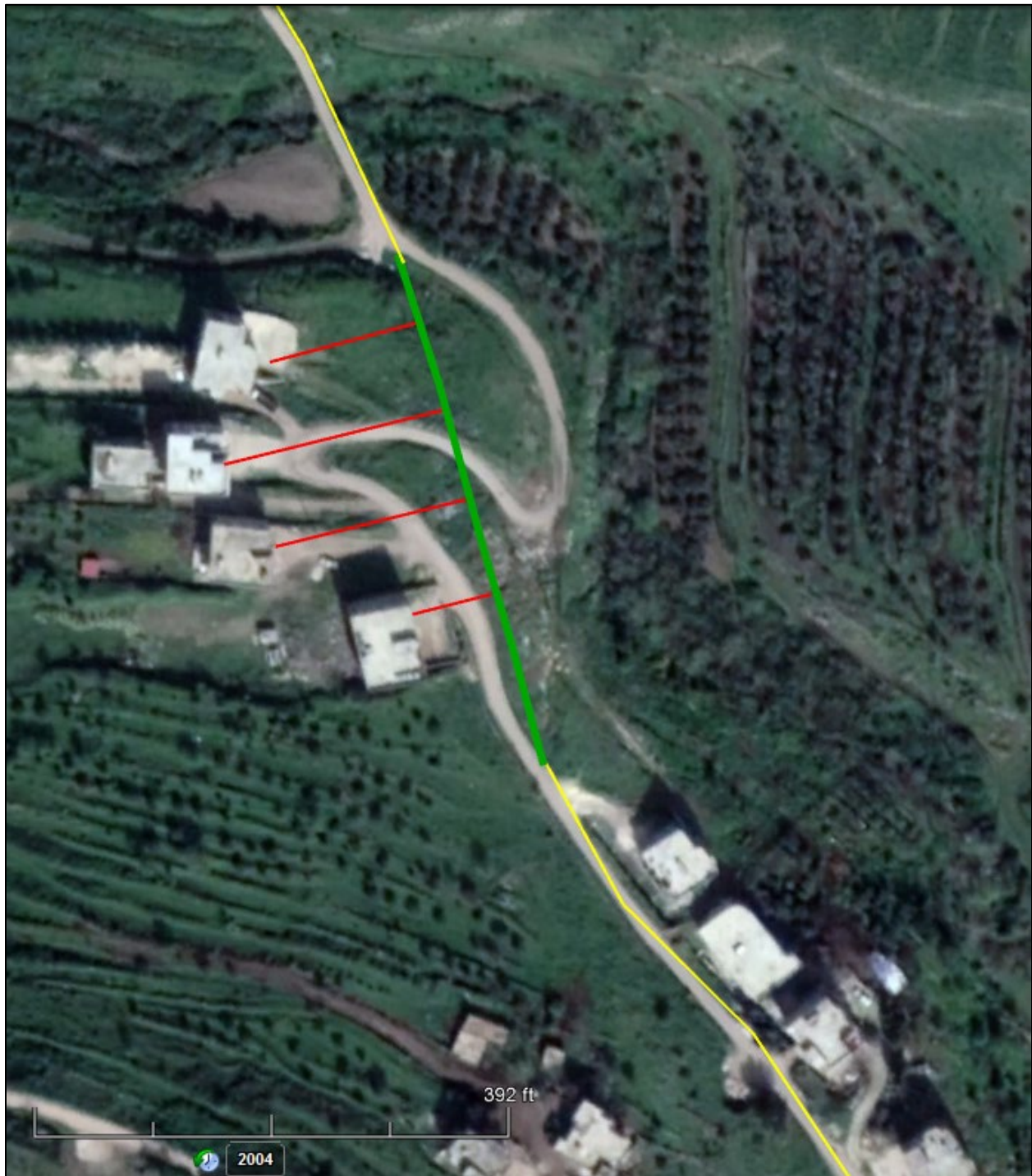
Figure 17-12 New 0.15km Segment of Asphalt Road
