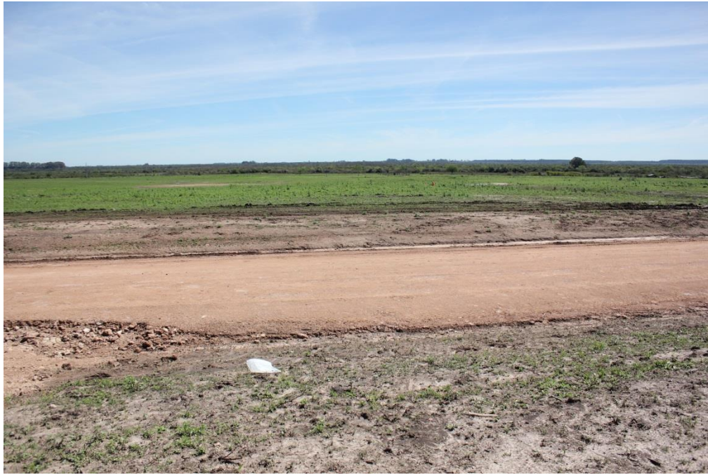
Figure 1: View of Raditon Site and initial construction activity
