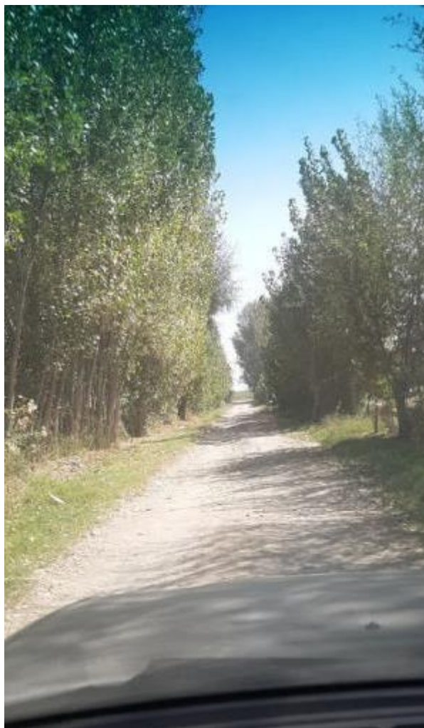
Figure 6-48. Road in Project Aol - 2
