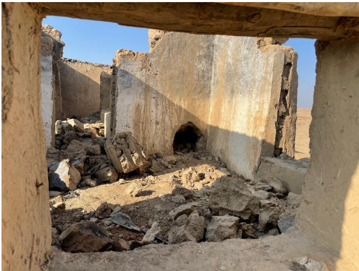
Figure 6-40. Inside of ruined Farm 5 house
