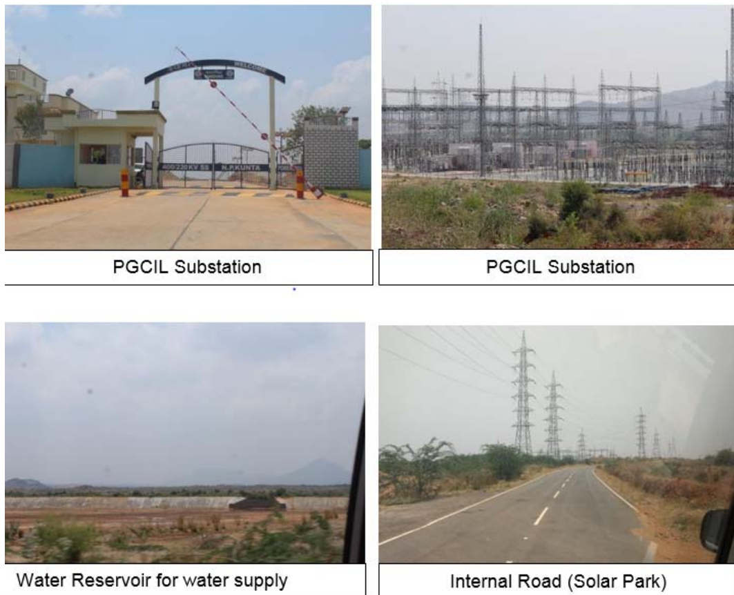
Figure 2.3: Existing Infrastructure within Solar Park
