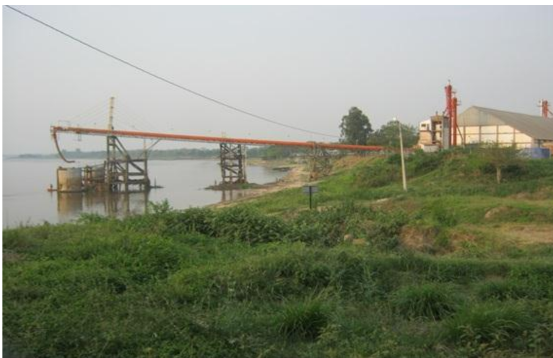
ANNEX VII: View to the existing port facility (Oct., 2012)
