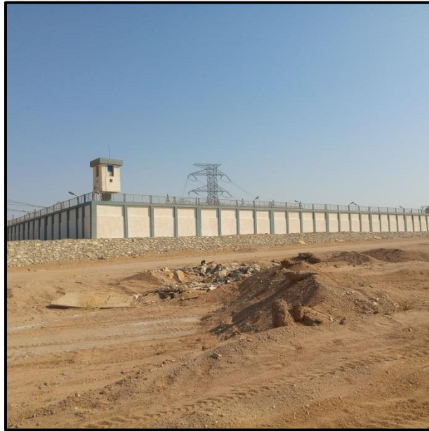
Figure 39: The Amunet Project Main Power Sub-station
