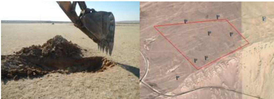
Figure 4-5: Trial pits
