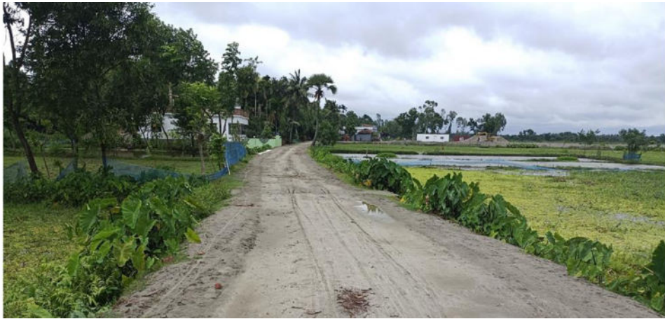
Access Road Development (ongoing)
