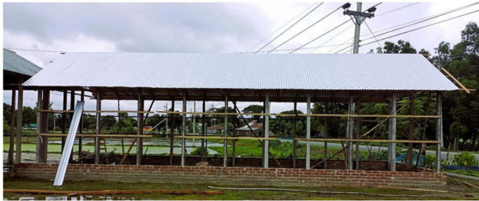
Temporary Storage and Labour Accommodation Development (ongoing)
