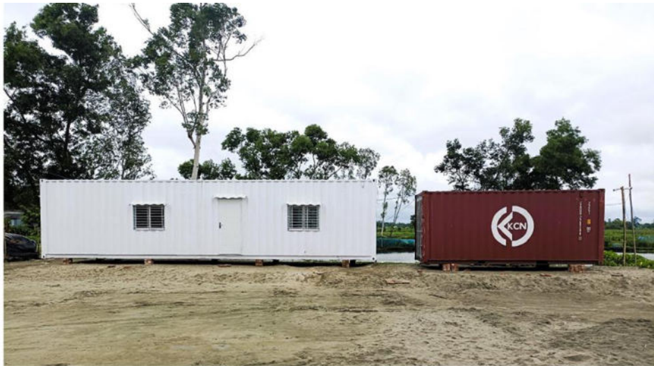
Site office Installment
