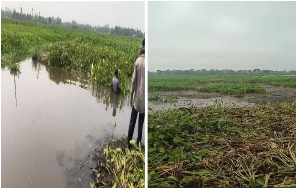
Site Cleaning (Water Hyacinth Removal)-Ongoing
