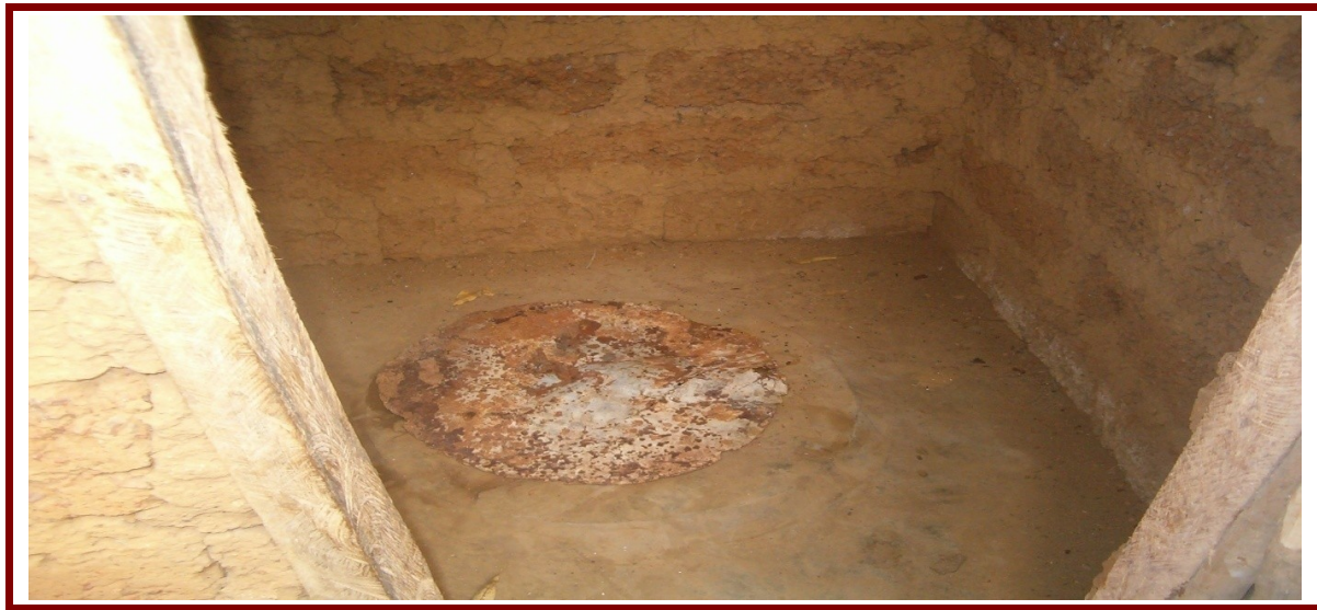
Plate 21: Typical open pit latrine
