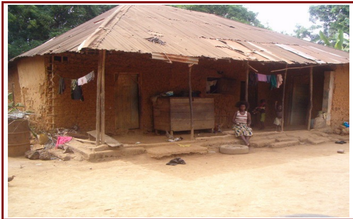
Plate 18: Typical village house constructed with mud and stick with corrugated iron roof
