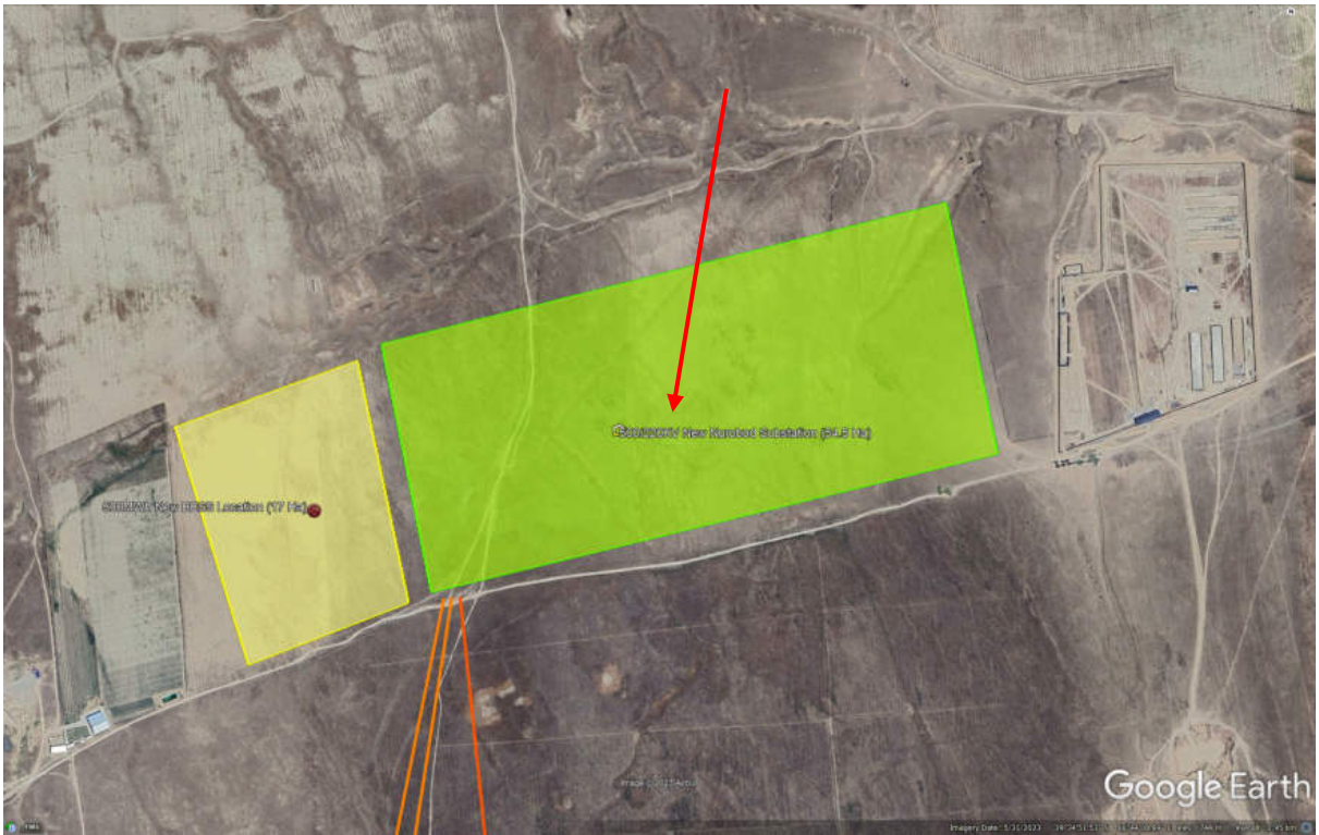
Figure 4: 500/220 KV Nurabad substation
