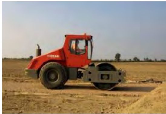
Figure 9: Preparing the land
