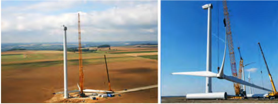
Figure 45: Fitting the rotor (formed by the hub, the cone and three blades).
