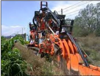
Figure 48: Machine for digging the trench about 1 m deep
