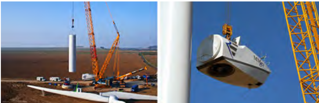
Figure 44: Assembling the nacelle
