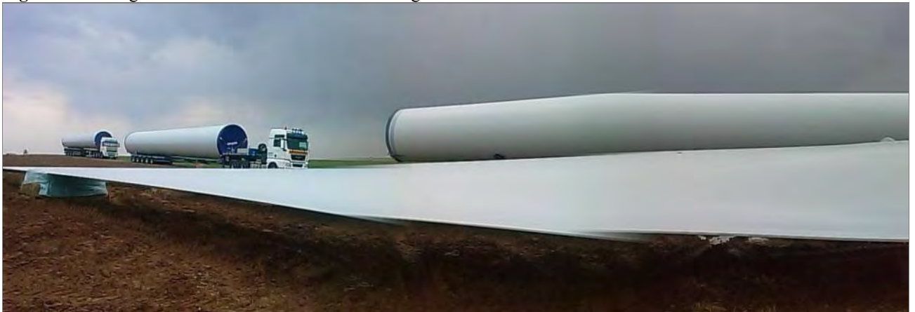
Figure 11: Storage of the blades on-site before hoisting them
