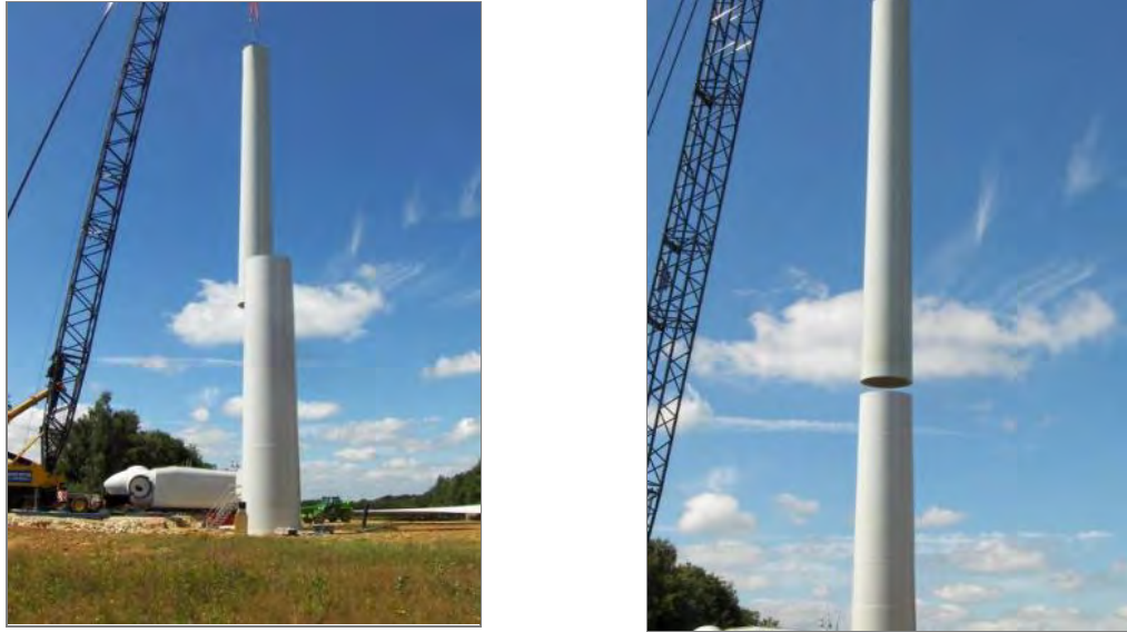
Figure 14: Mounting the tower's components
