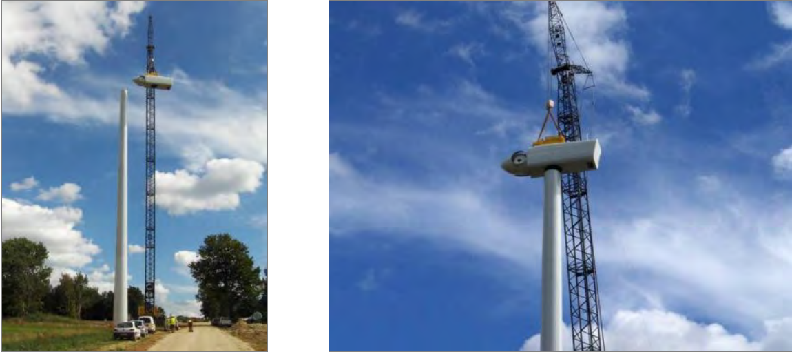
Figure 16: Mounting the nacelle on the tower
