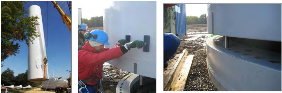
Figure 13: Mounting of the first component of the tower
