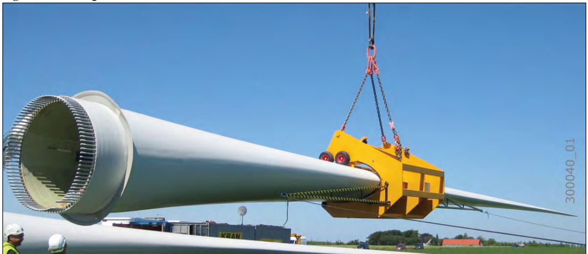
Figure 17: Lifting a blade
