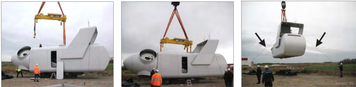
Figure 15: Preparation of the nacelle
