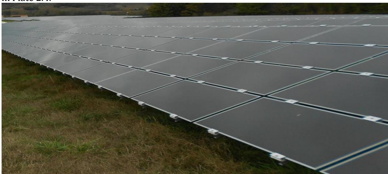
**Plate 2.4: Typical Appearance of Thin-Film CdTe Arrays**
