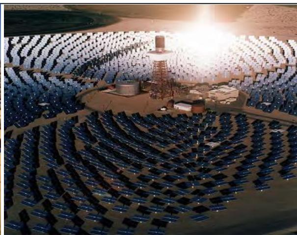
Plate 2.2: Typical Power Tower Facility
