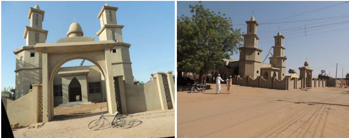
Figure 4.23: The Newest Major Mosque in Kankiya
