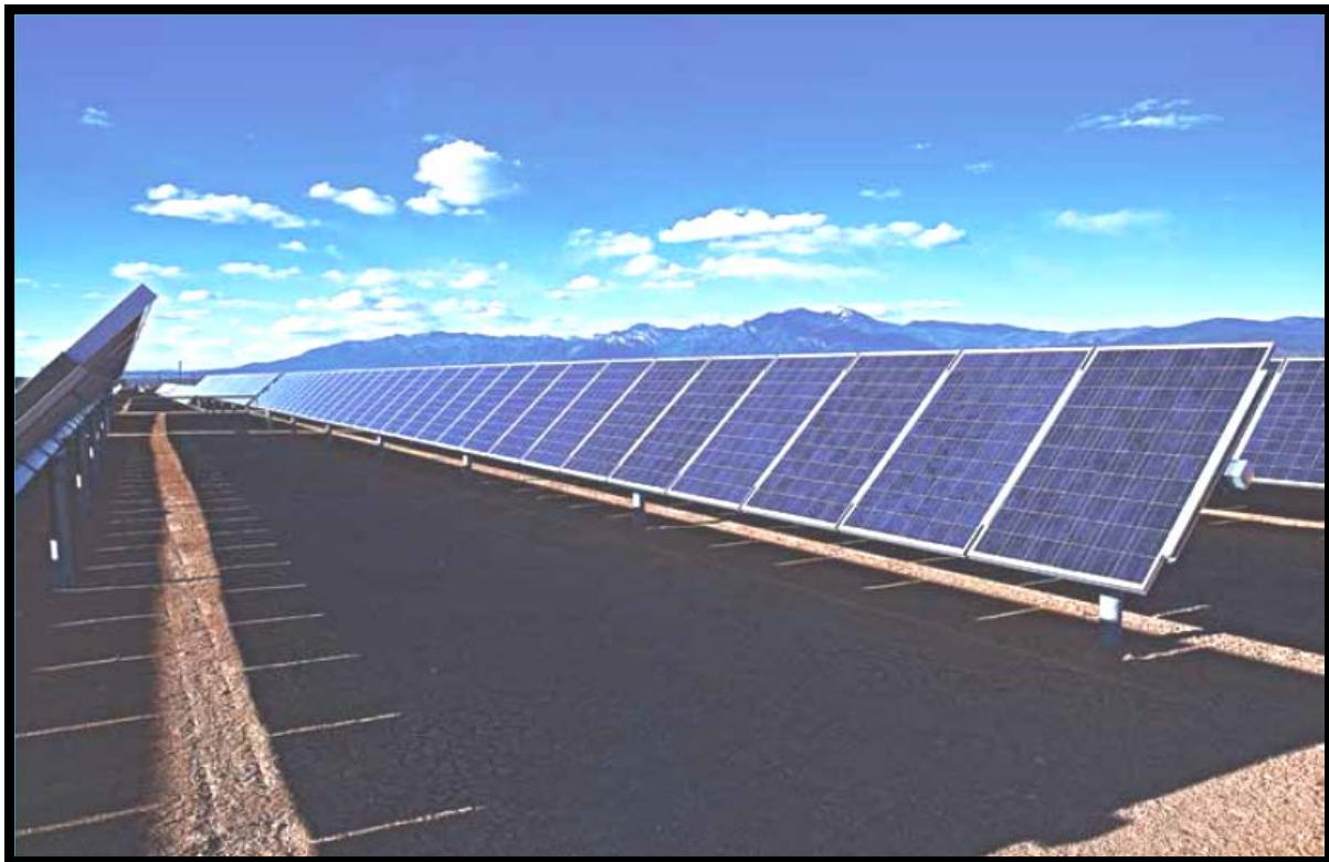
Figure 3.21: Spacing Between Module Rows
