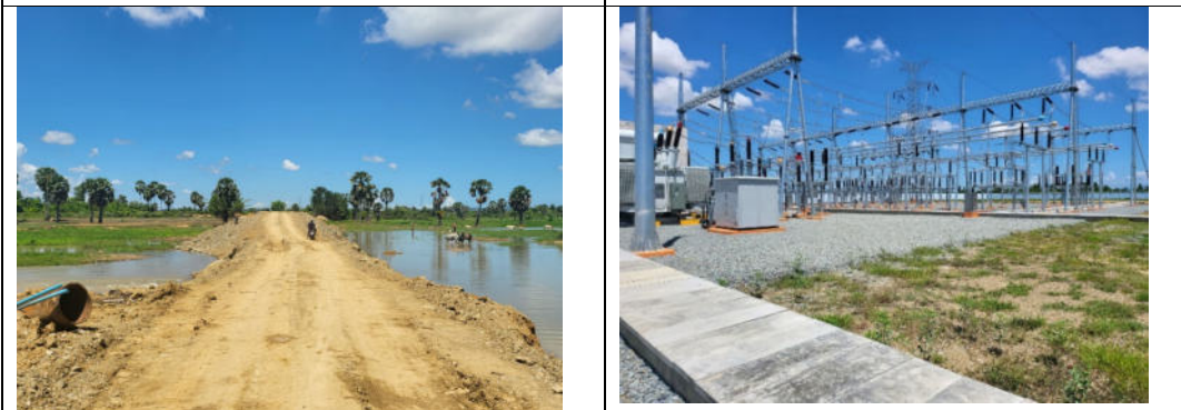
Site inspectors by PMO1 and PIC (23 June 2023)
