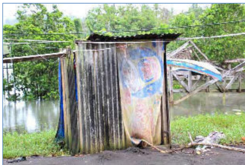
Figure 8-11 Emergency Toilet is made of Recycled Materials
