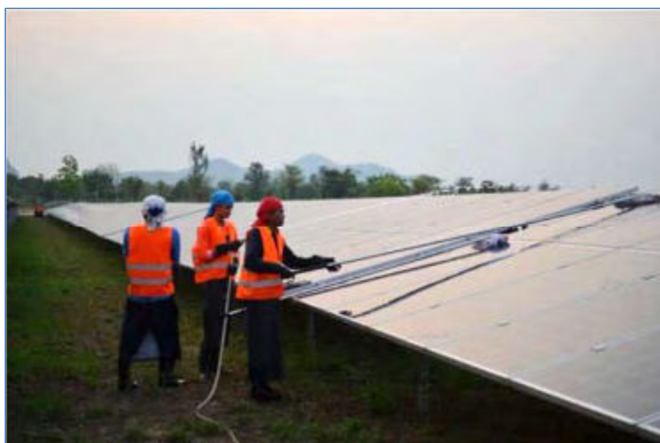
Figure 2-10 PV Module Washing
