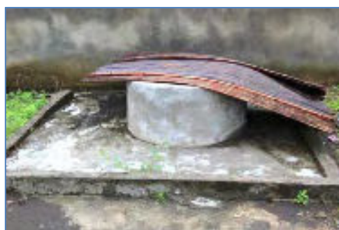
Figure 8-10 A Dug Well
