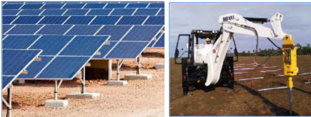
Figure 2-9 PV Module Foundation Establishment
