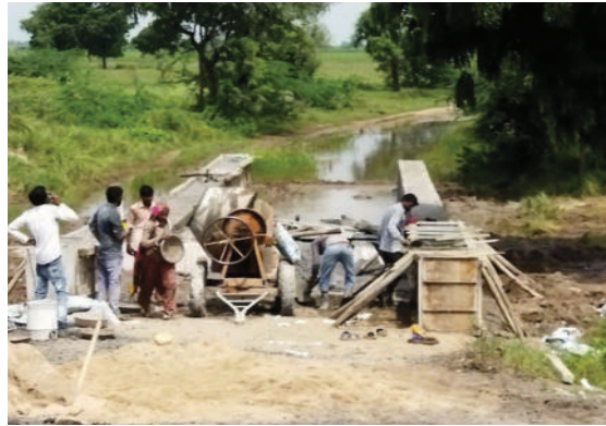
Access road towards project site (Funded by Village Panchayat)
