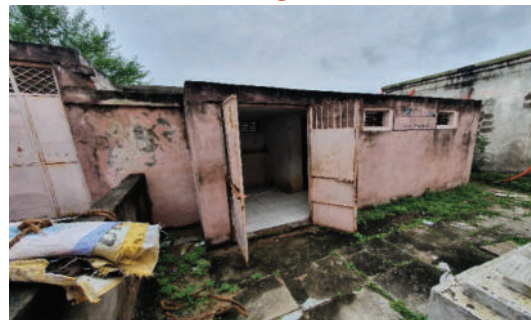
Toilet facility, Jakhan PS
