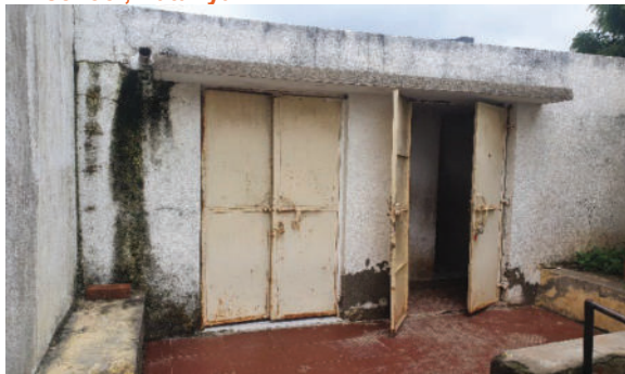
Kitchen Facility, Katariya
