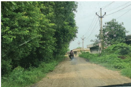
Approach road towards Jakhan village
