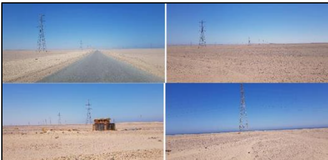
Figure 78: Overhead Transmission Line (OHTL) in the Project Area
