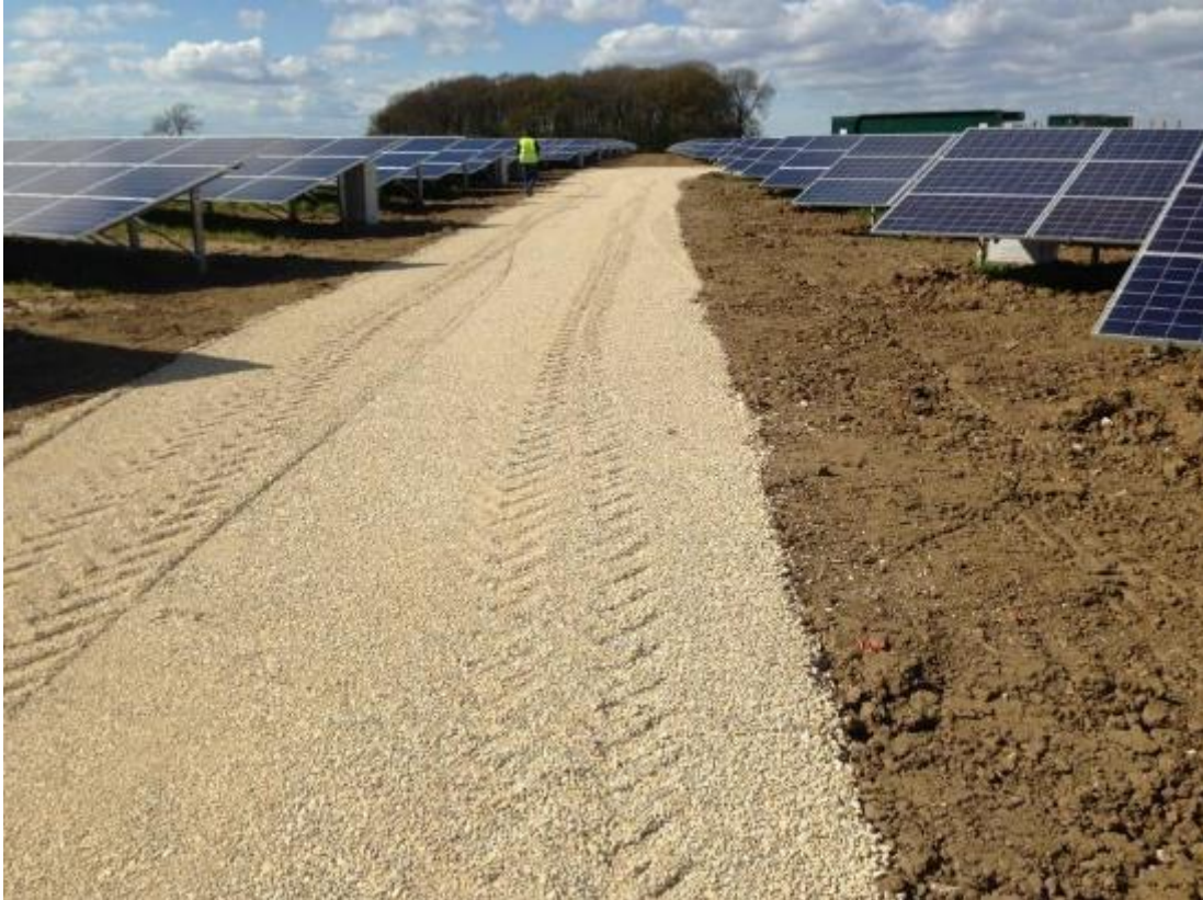
Figure 2-14: Typical internal access track
