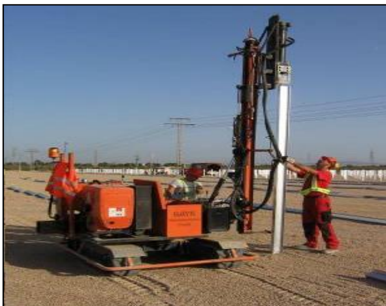
Figure 2-9: Hydraulic Driving Machine for Installing Piles
