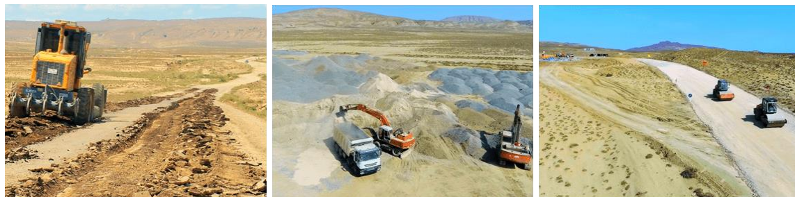
Figure 11-4: Ongoing construction works of the new road “Gobustan – Volcanoes
