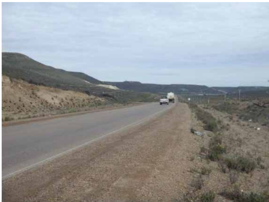
Figure 34. View of Provincial Route 12.
