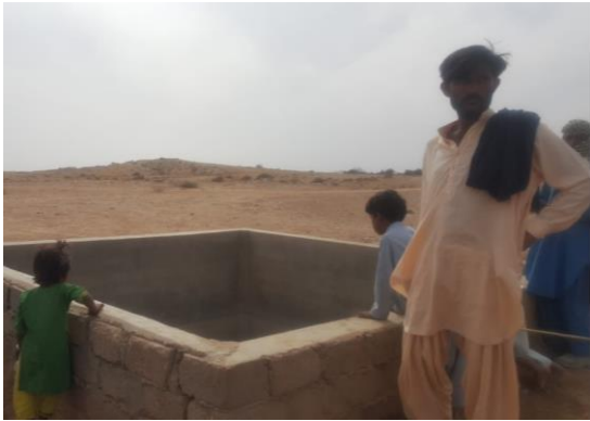
c. Concrete water storage tank
