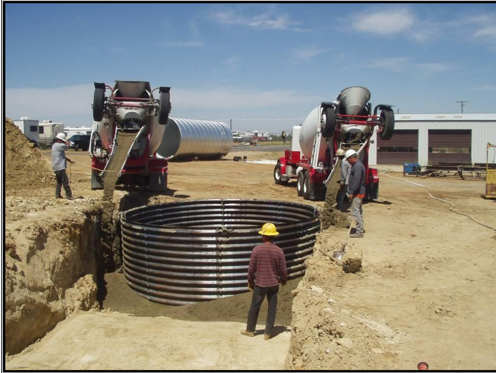
Figure II.9. Example for installing a pier foundation.
