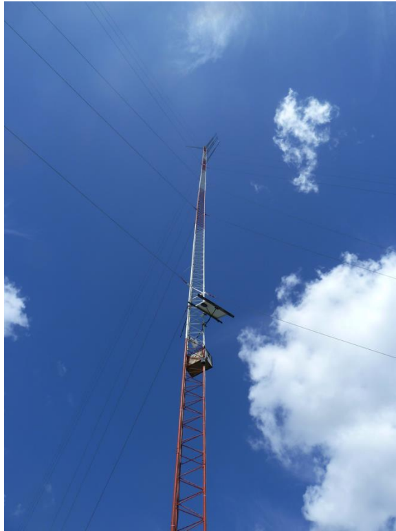
Figure II.10. Typical meteorological tower with single pole and metal straps.
