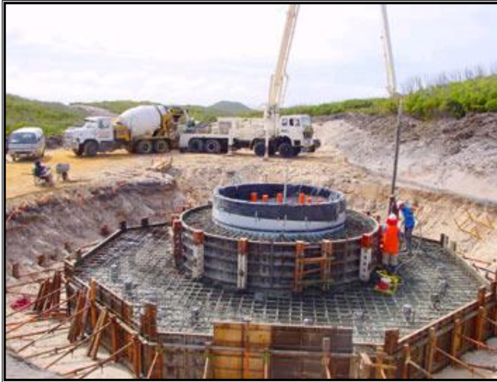
Figure II.8. Example for installing a mat foundation.
