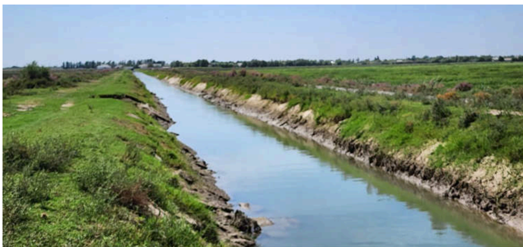
Figure 9: Irrigation canal in Syrdarya region
