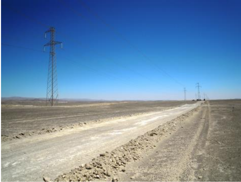
Figure 1: Project area- view to north and access road
