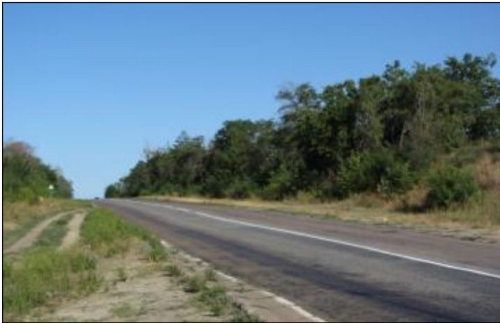
Fig.2.1. Hedgerows along the bypass road and 330 kV OTL route
