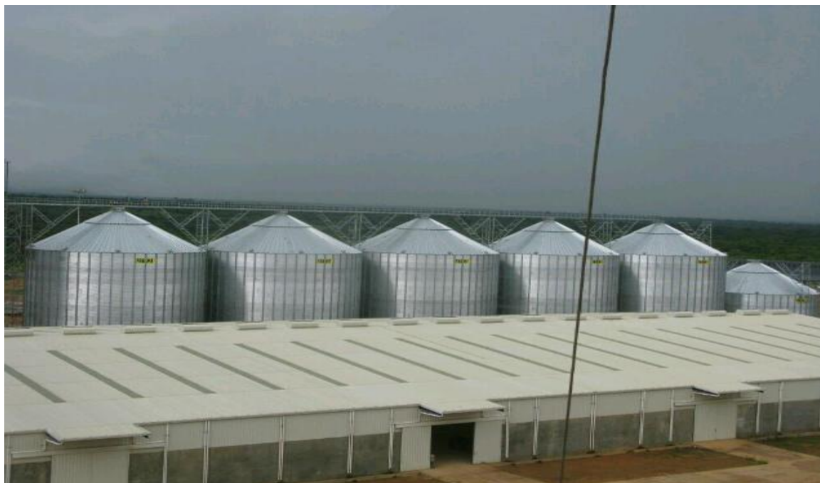
Figure 4-4: Maize storage facilities at AMCC
