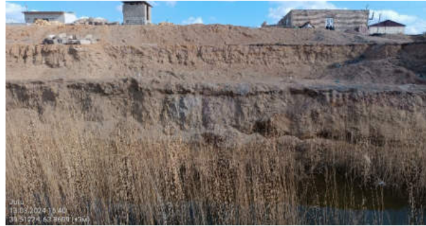
Figure 34. Waterbody along the access road
