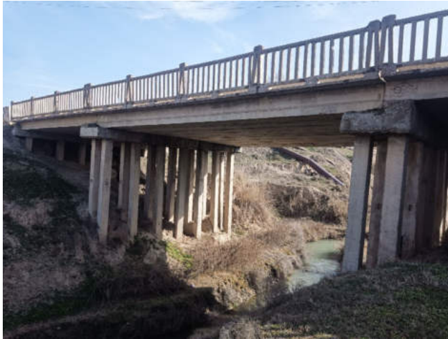
Figure 24 Bridge over the canal
