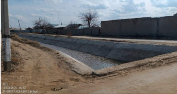
Figure 33. Canal near the access road
