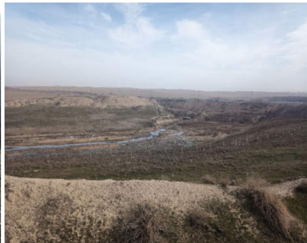
Figure 15: Drainage under the railway «Afrosiab» with no access
