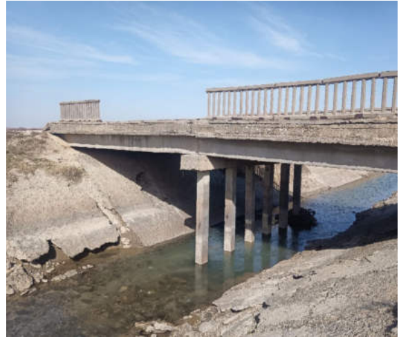
Figure 25: Bridge over the canal
