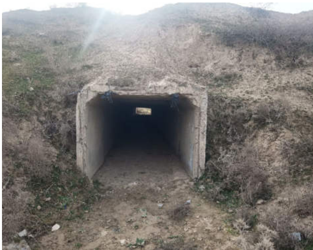
Figure 26 Drainage under the car road
