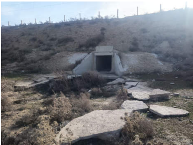
Figure 14: Drainage under the railway «Afrosiab»
