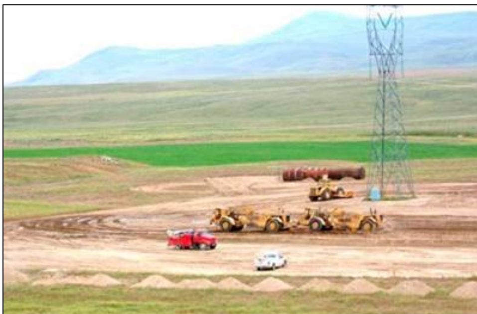
Figure 7-2: Site preparation for construction of typical sub-station
