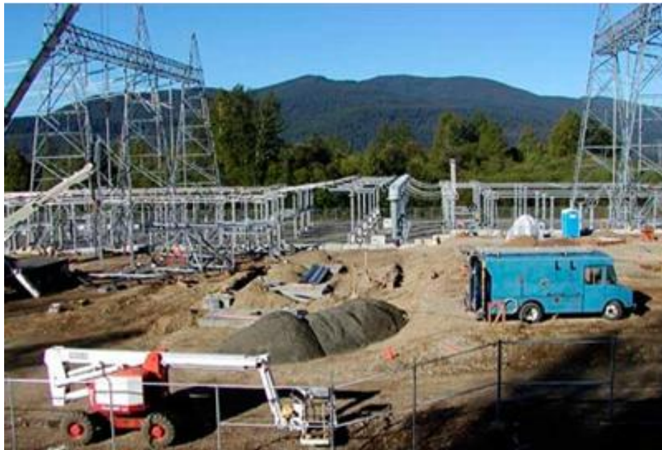
Figure 7-9: Sub-station under construction
