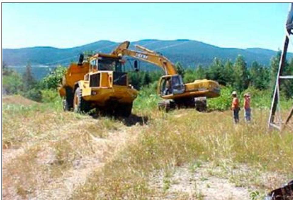
Figure 7-1: Image showing clearing of vegetation in hilly terrain
