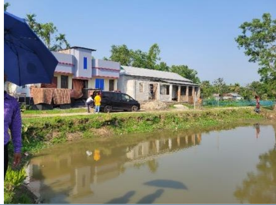
Residential Area near north side of the project area
