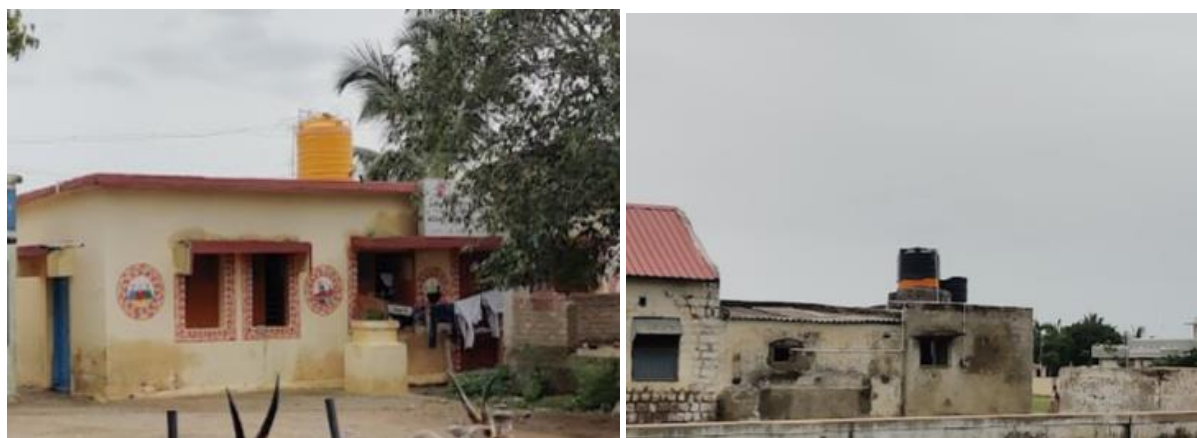
Figure 6.30 Overhead water storage
