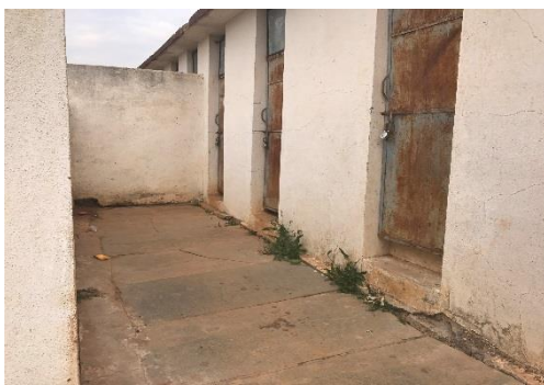
Separate toilet arrangements at Upper Primary School, Veligallu
